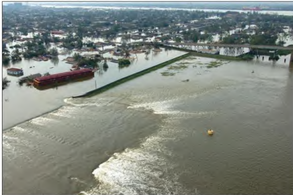
Figure 1-8. Aerial view of damage to one of the levees caused by Hurricane Katrina (photo taken on August 30, 2005, the day after the storm hit, New Orleans, Louisiana).
