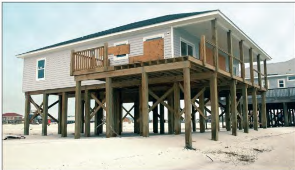
Figure 2-5. Successful pile foundation following Hurricane Katrina (Dauphin Island, Alabama)
