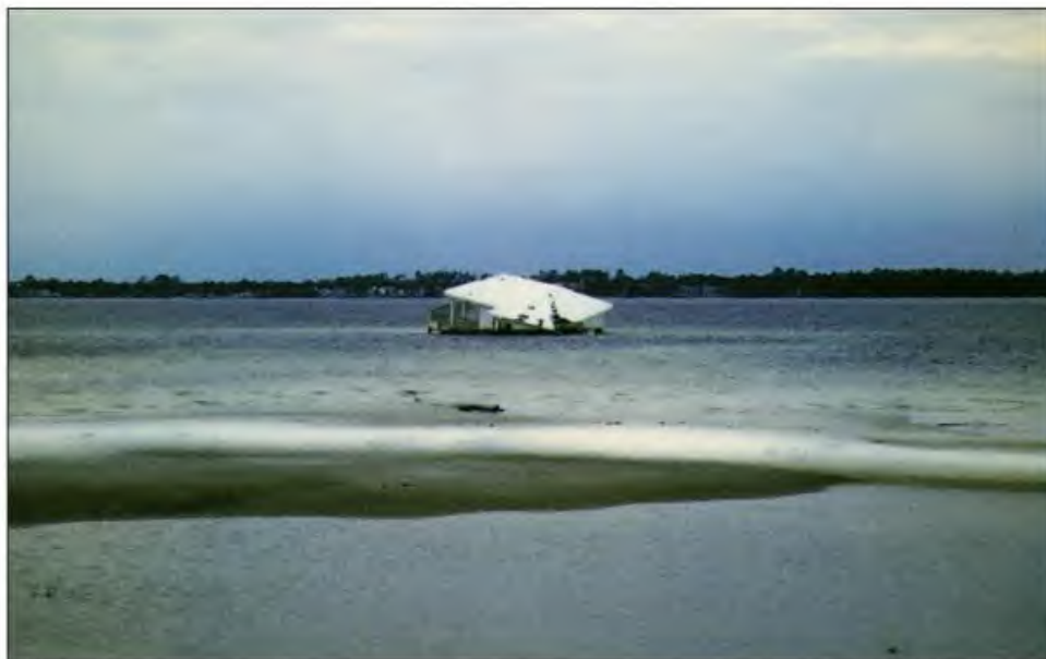
Figure 1-9. During Hurricane Opal (1995), this house was in an area of channeled flow between large buildings. As a result, the house was undermined and washed into the bay behind a barrier island.
