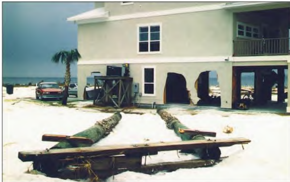
Figure 1-12. Pier piles were carried over 2 miles by the storm surge and waves of Hurricane Opal (1995) before coming to rest near this elevated house in Pensacola Beach, Florida.
